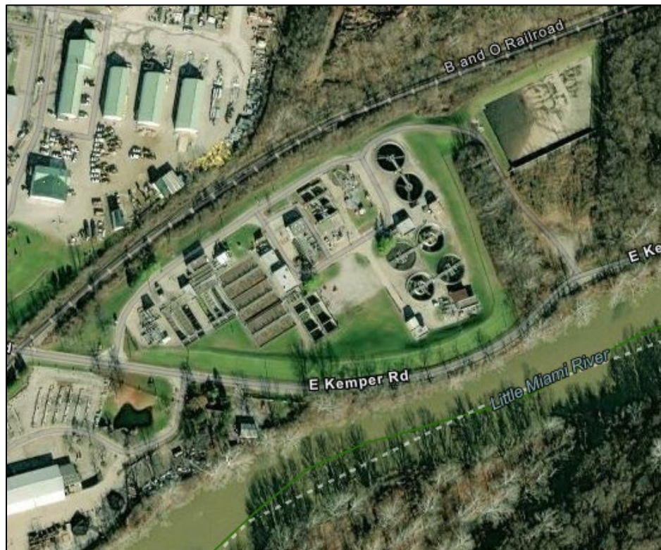
Figure 2. Polk Run WWTP
